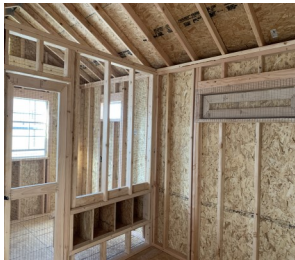
Available— Interior Wire Partition Dividing Nesting Area to Create Feed Storage
